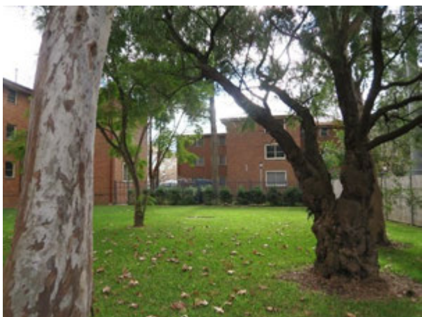
Picture 7 – Southern elevation of walk-up flats at 247-251 Cope Street, facing north from McEvoy Street
