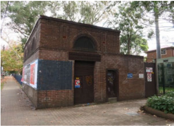
Picture 23 – Privately owned and locally heritage listed sub-station fronting McEvoy Street (address being 336 George Street)
