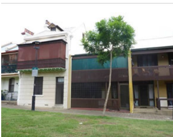
Picture 75 – Terraces along Forbes Street, designed a simple referential style
