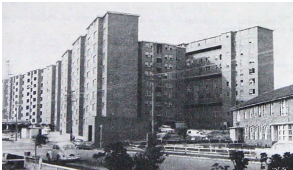
Figure 107 – McKell Place under construction, c. 1962-93
