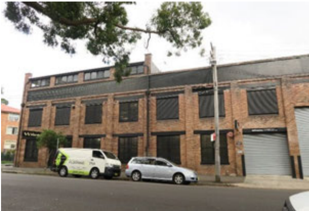
Picture 17 – Privately owned commercial warehouse building at 116 Wellington Street
