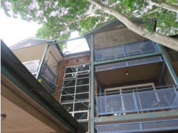
Picture 3 – Eastern elevation of one of three of the first blocks, as viewed from George Street
