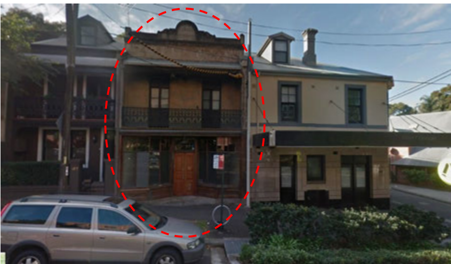
Figure 33 – Terrace house/shop, Pitt Street elevation.
