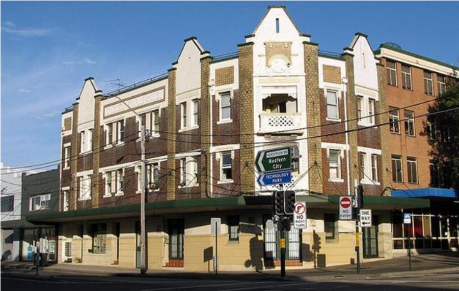
Figure 32 – Cricketers Arms Hotel, Henderson Road elevation.
