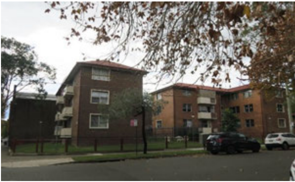
Picture 9 – Typical walk-up buildings at 6-8 John Avenue
