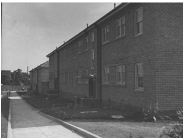
Picture 61 – View of two of the blocks, facing south on Swanson Street
