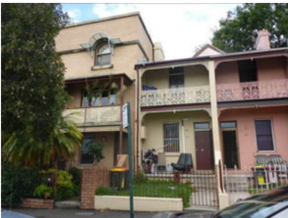
Picture 81 – Terraces along Phillip Street, featuring referential parapets, arched windows and overall form in a contemporary style. Victorian terraces shown at right of frame
