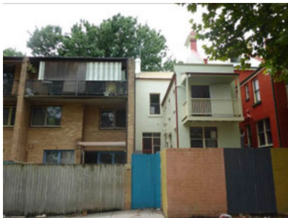
Picture 74 – View from the central courtyard located at the corner of Cathedral and Dowling streets, showing the rear of properties located on Dowling Street (contemporary on left and Victorian to right)
