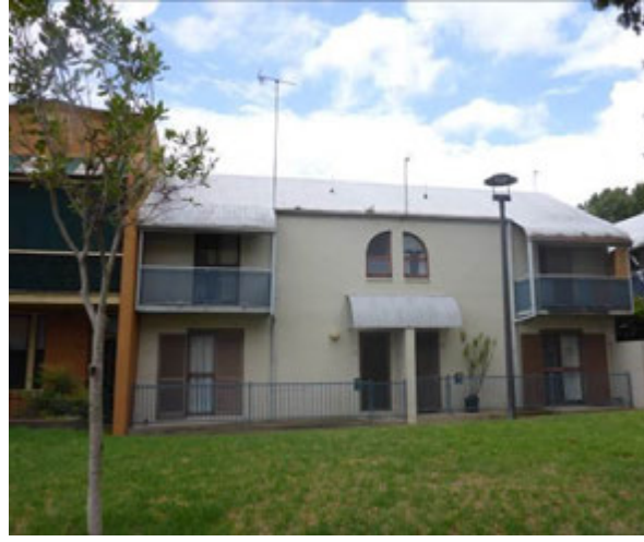
Picture 78 – Terraces along Forbes Street, featuring referential arched windows and overall form in a contemporary style
