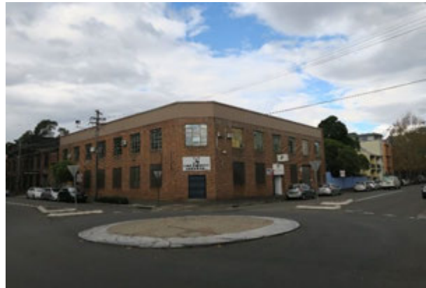
Picture 18 – Privately owned commercial warehouse building at 221-223 Cope Street
